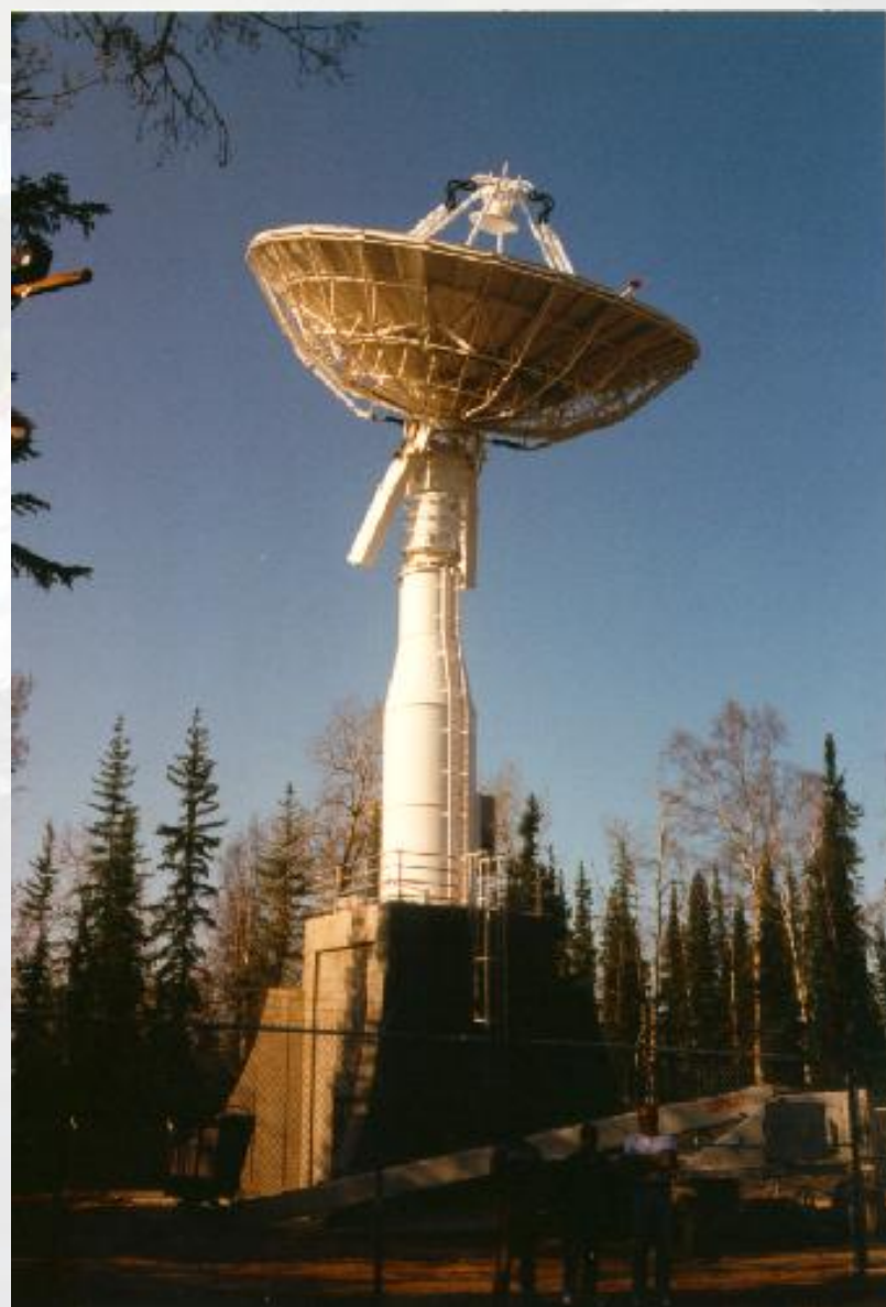
Alaska SAR Facility 11 meter antenna
