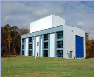
Cargo Processing Bldg
