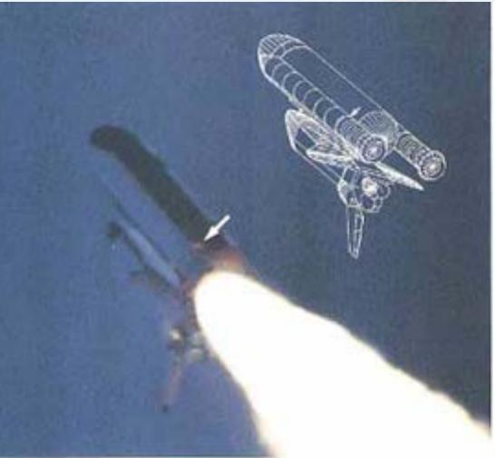
At 58 781 seconds, the feet ficker of fame appeared, flatery visible above, it grew end a large plume and becaus is impinge on the External Tark at about 60 seconds. Flame is give ported in the computer drawing between the sight boostor and the tark, as in the case of particisincke public. At far sight larged, sight is seen escaping from the according towershell become Tark.
