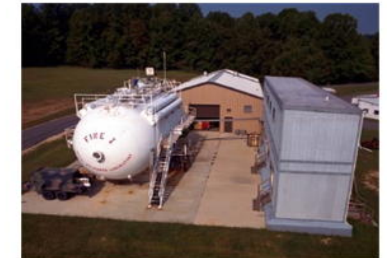
Submarine Fire Facility
